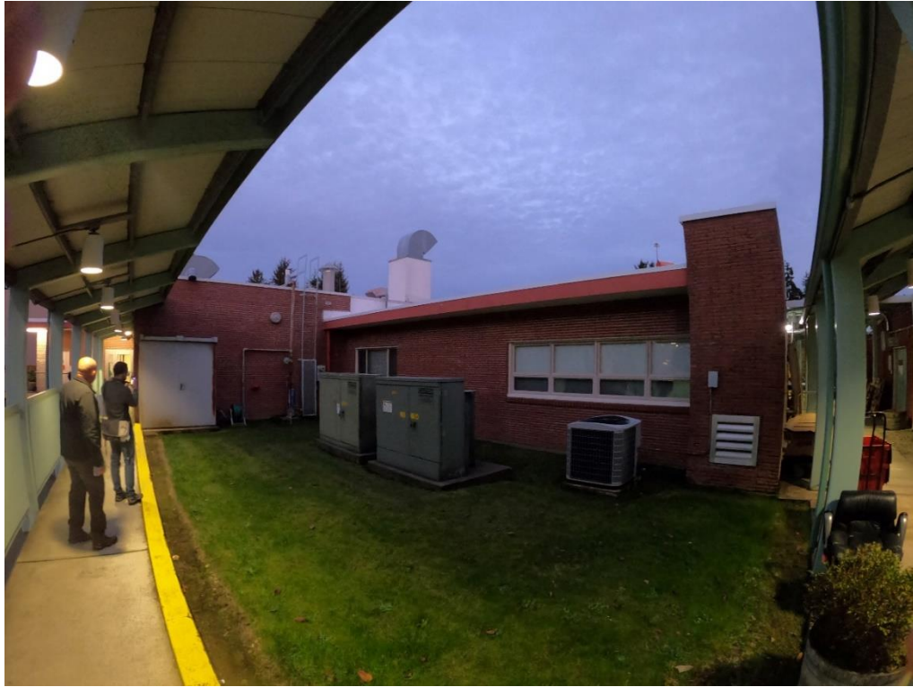
Boiler Room and Original Hospital at Southeast Corner
