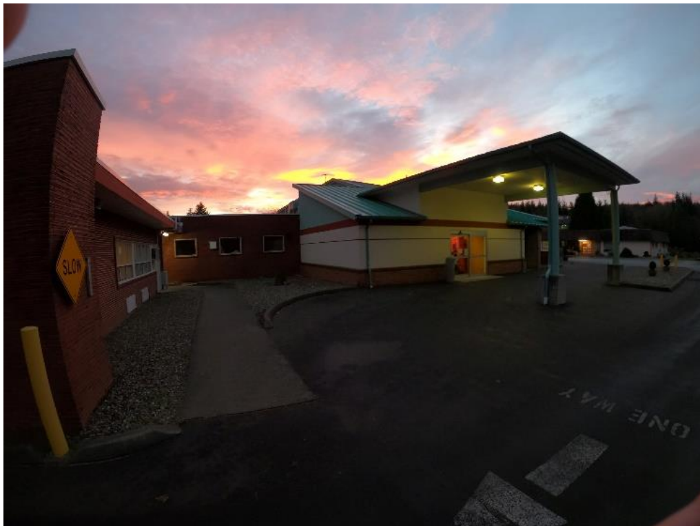
West View of Original and 1999 Hospital Addition
