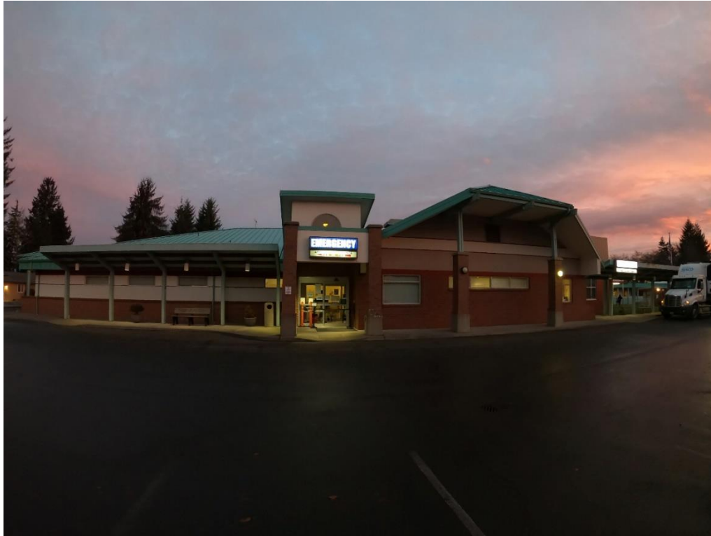
Front Entry of 1999 Building Addition
