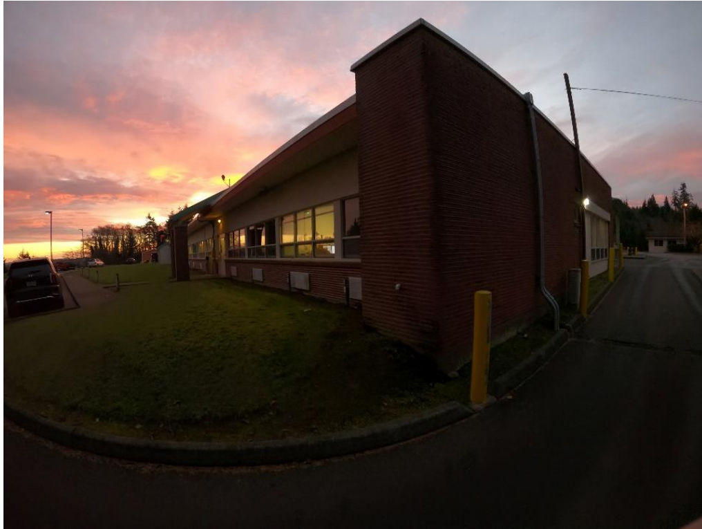
Original Hospital North and West Wall Exterior
